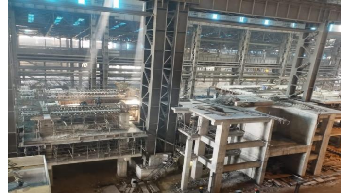
Ladle Turret & Casting Platform at SMS2, BPSL Phase II
