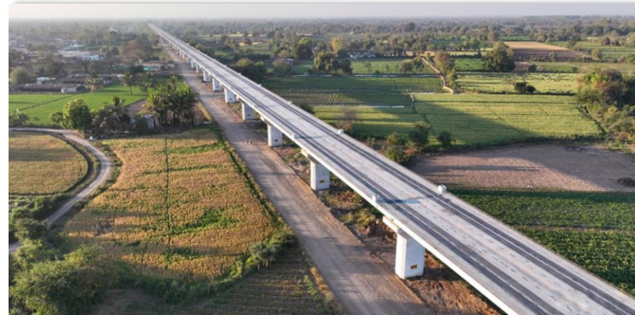
MAHSR Viaduct at Anand District, Gujarat
